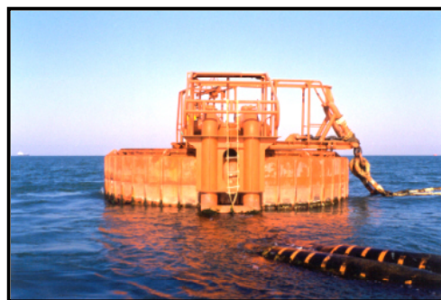
Fig. 28 - Single Point Mooring of Indian Oil Corporation near Vadinar
