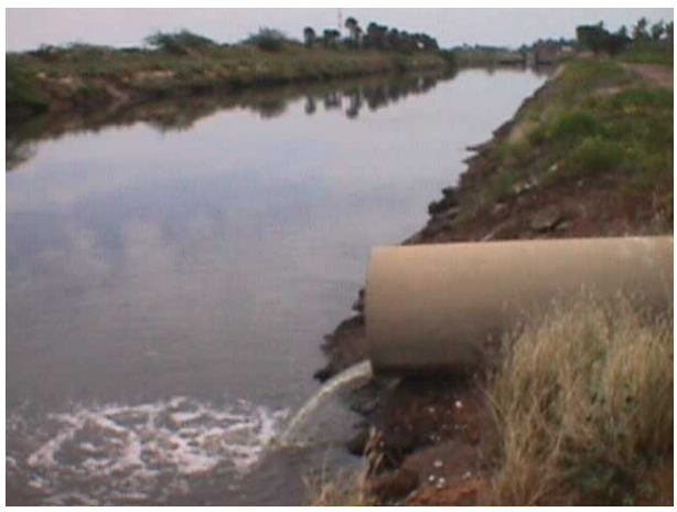
ONE OF THE NON POINT WASTEWATER DISCHARGE FROM INDUSTRIAL SOURCES
