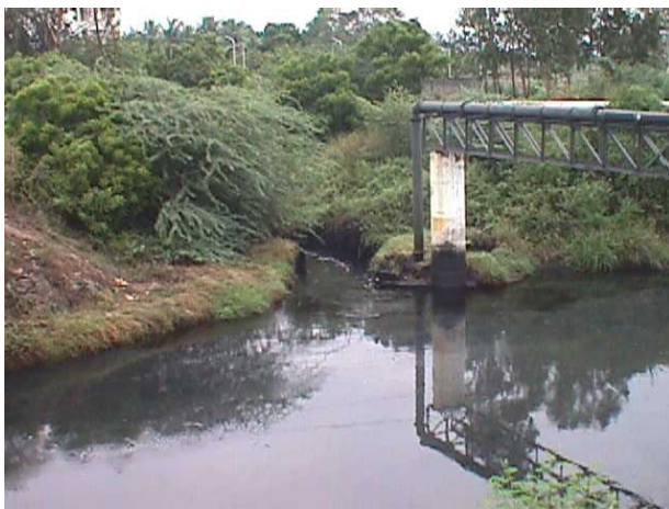
MRL OILWASTEWATER DISCHARGE (WITH OIL)
